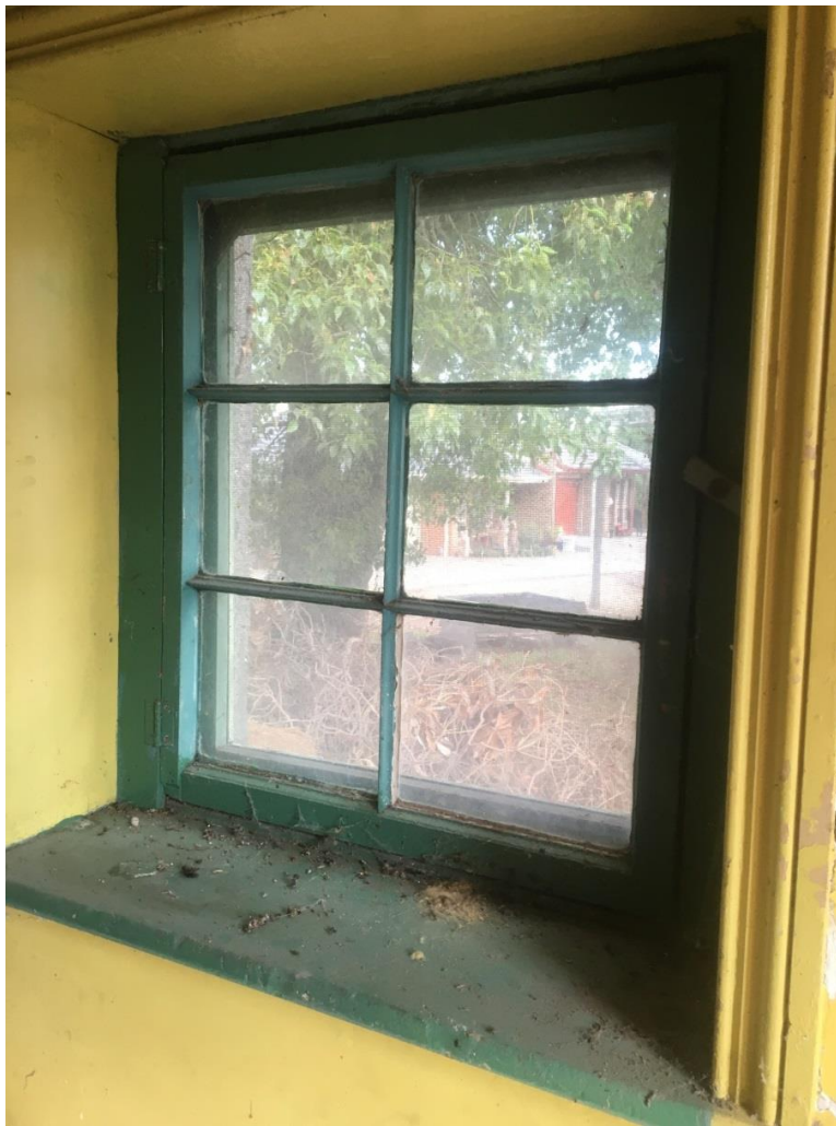
Figure 18: Victorian-style window with 'lamb's tongue' profile glazing bars on the south side of the outbuilding (source: Context 2016)
