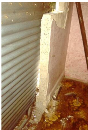
PHOTOGRAPH OF MONOLITHIC REINFORCED CONCRETE WALL WITH FLARED BASE, 36 KING STREET, NORTH FITZROY (SOURCE: PAUL ROSER, 'CONCRETE HOUSES')
